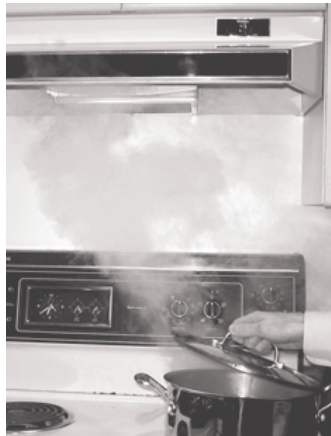
Use your kitchen exhaust fan or range hood to remove humidity generated by cooking. The exhaust fan should be vented to the outside.
